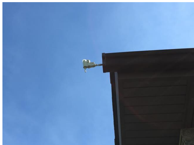
PROPER INSTALLATION OF A RAIN SENSOR
