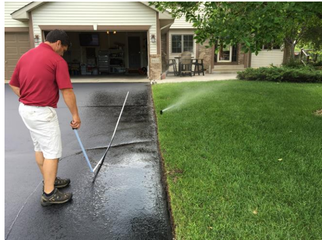
IMPROPERLY ADJUSTED SPRINKLER
