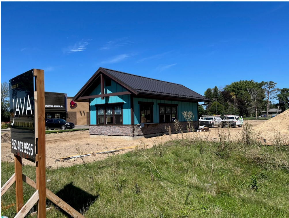
New Caribou Drive Through Under Construction
